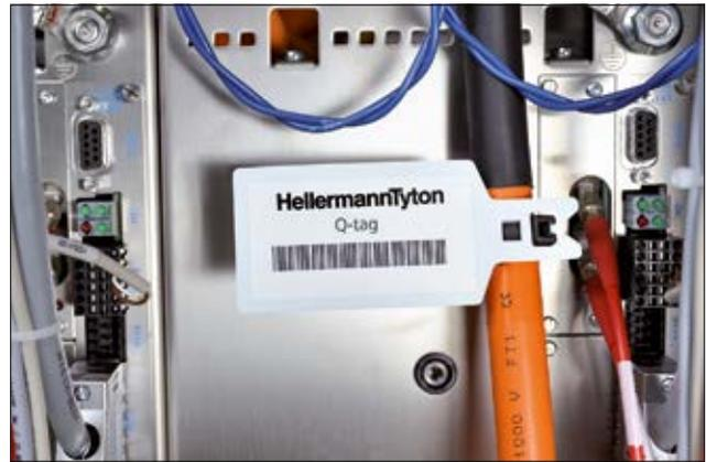
The flagged orientation of Q-tags ensures that printed texts are easily visible.
