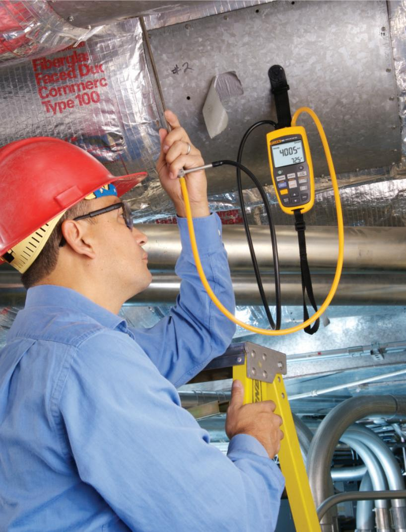
Using the Fluke 922 low pressure differential meter in a duct traverse.
