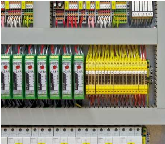
Scalable safety relay solution with PSRmini
