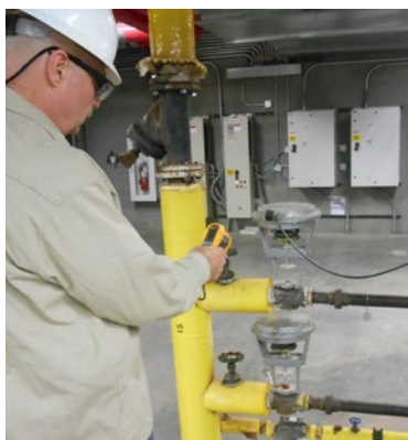
Measuring the steam temperature at the inlet to the humidifier valve.
