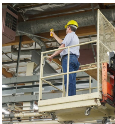
Identifying the temperature of ceiling-mount equipment.
