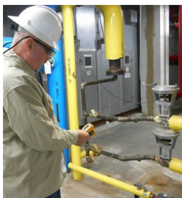
Testing the steam trap to see whether the trap has failed open and is wasting steam.
