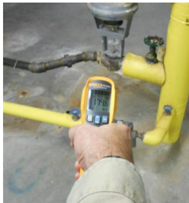
Viewing the temperature of the condensate line from a steam trap, to make sure it is functioning properly.
