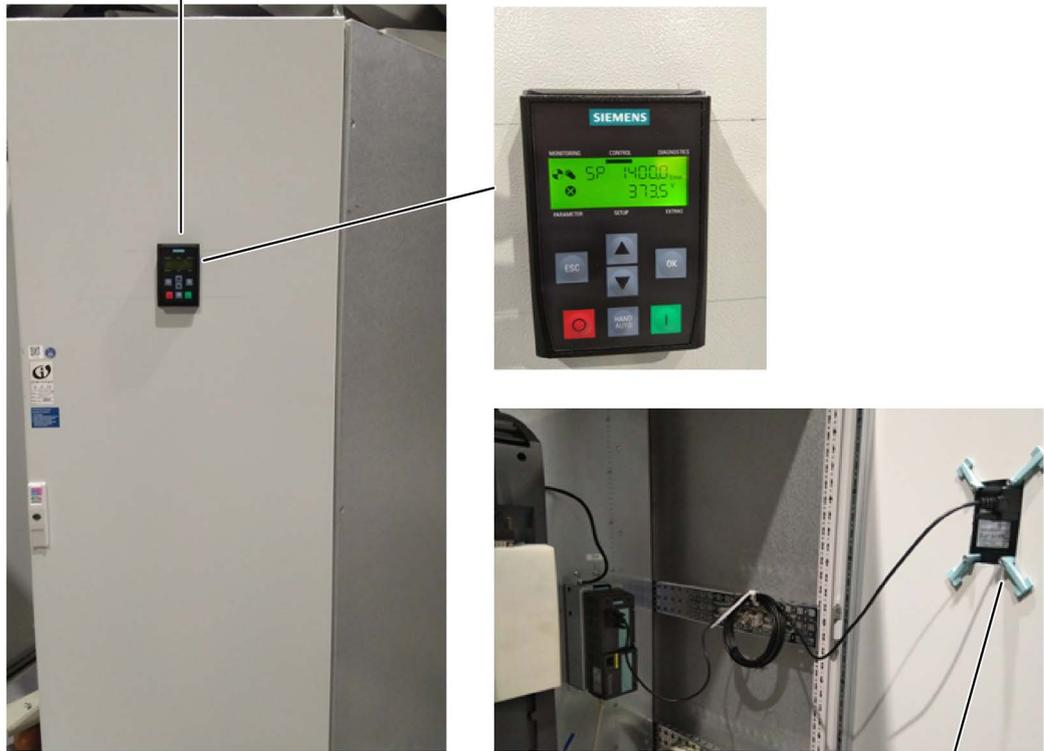
Fastened using the door mounting kit
