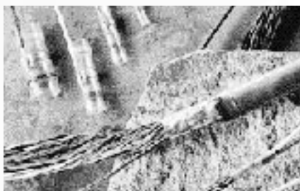
Terminating ground wire to cable shield
