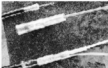
Terminating coaxial cables
