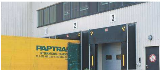
Numbered Panels: Loading Dock Panels, Gangway Panels, Bin Panels
