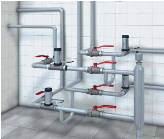
Control positioning of valves in the processing systems of dairies or breweries.
