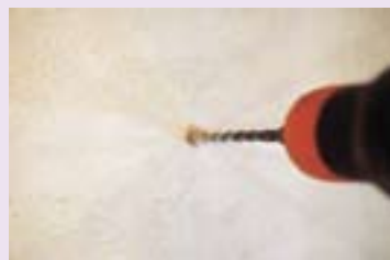
Drill to diam. 8 mm
