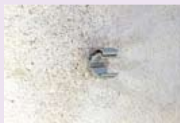
Conduit support is fixed
