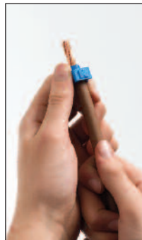
Push Smart meter collar onto cable.
