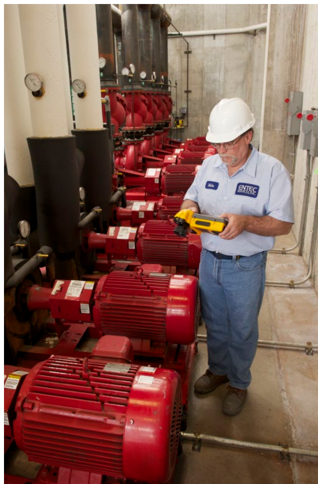
Mike Schum uses a Fluke Ti45FT Thermal Imager to compare performance across an array of motors and pumps. Next to Mike, the chilled water pumps move chilled water to and from the air handling units located throughout the hospital. Behind him, the uninsulated condenser water pipes move condenser water to and from cooling towers.
