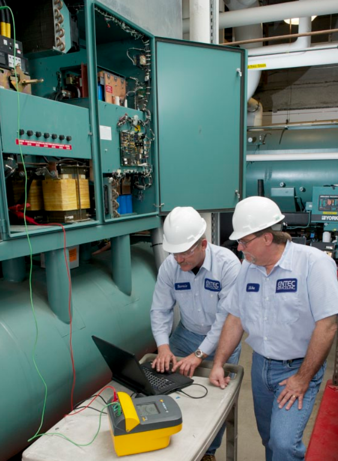
Bernie Kargol (left) and Mike Schum download and discuss data from the Fluke 1555 Insulation Resistance Tester after running tests (when the chiller is powered off) on one of several chillers at a large hospital.
