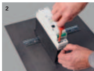
2 Connect mains and motor cables.
