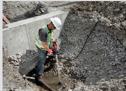
Push Water Out of Trenches, Basins, and Over Walls with 4.5M Max Head Height
