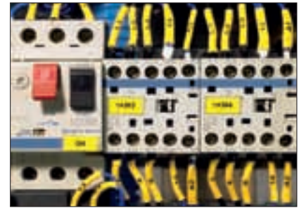
High performance halogen free printed markers after shrinking
