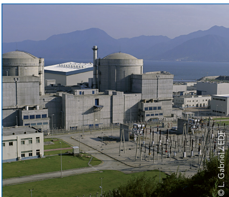
Class 1E Safety Equipment
