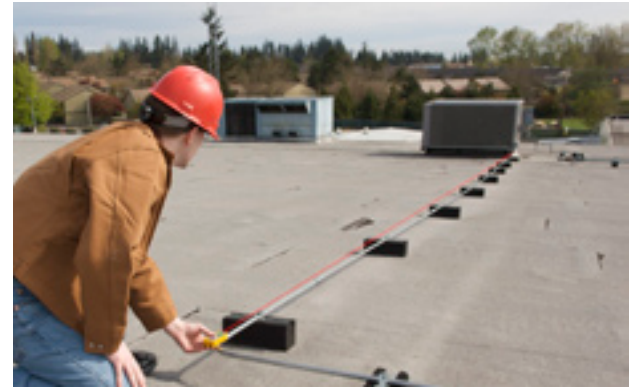
Measuring long conduit runs.
