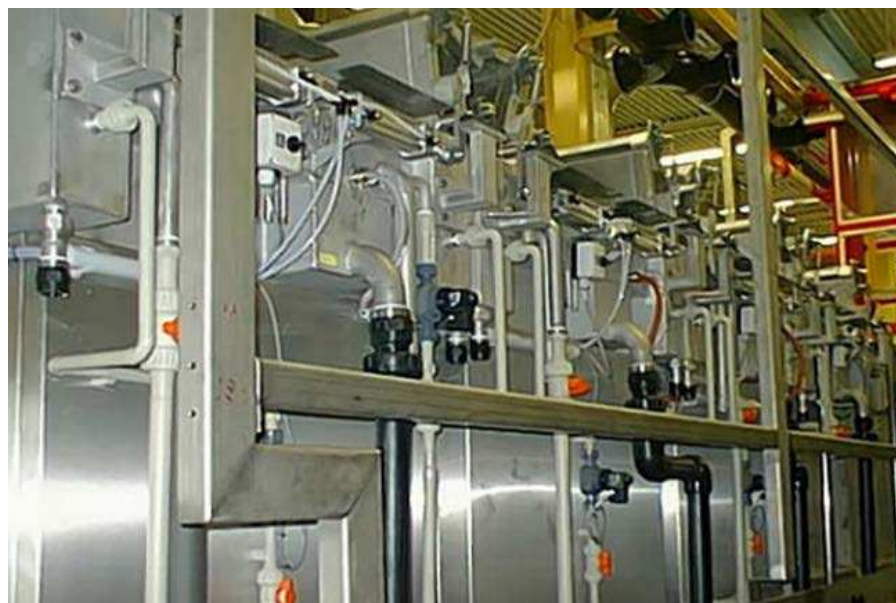
Phosphating plant at SKF
