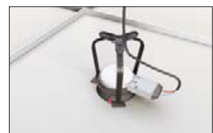
4. Connect the downlight to the power supply and fix the cable into the routing eyelet.
