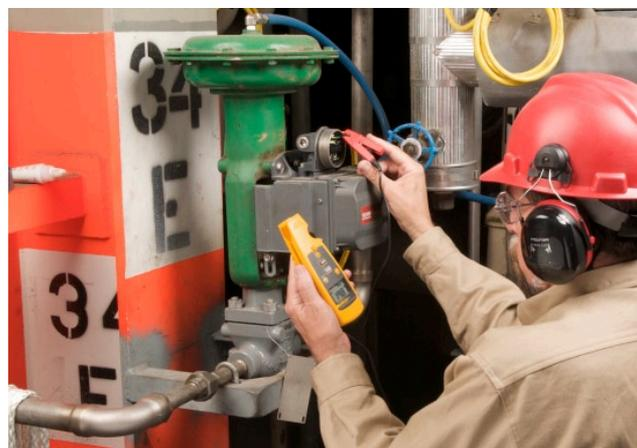
Checking a Fieldvue control on a Fischer valve for a condensate collection system.
