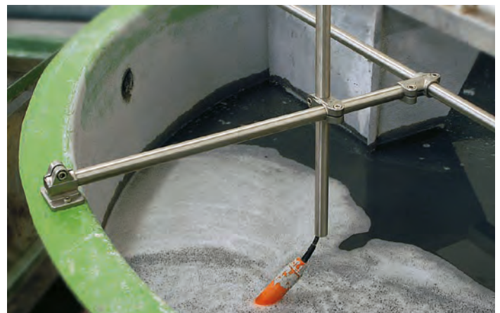
Simple probe fixation in an aggressive environment
