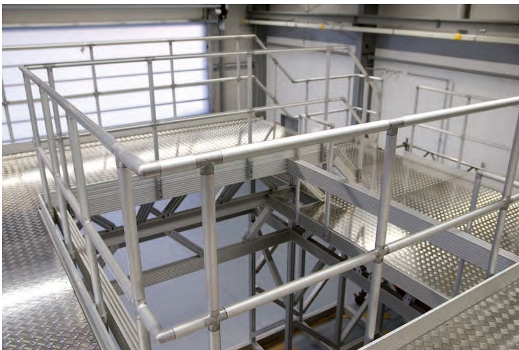
Working platform with ITAS railing
