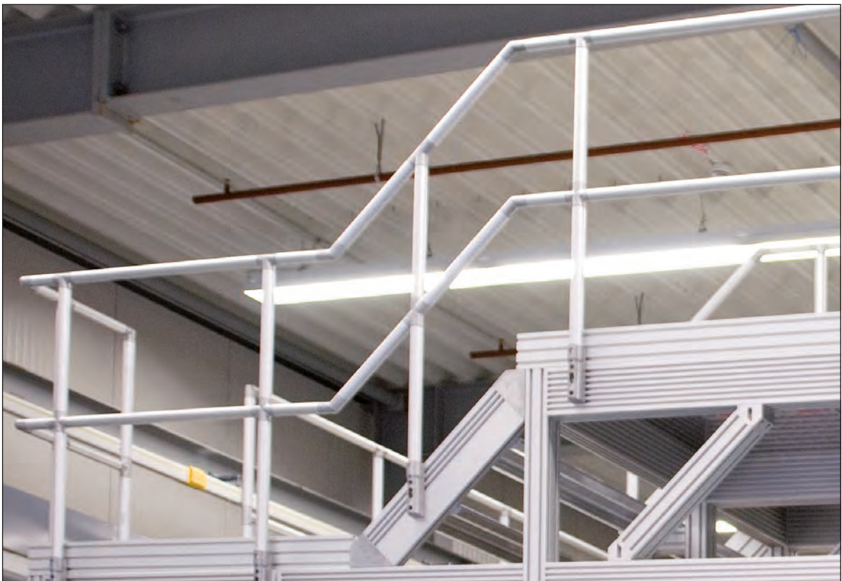
Staircase between two operating platforms.
