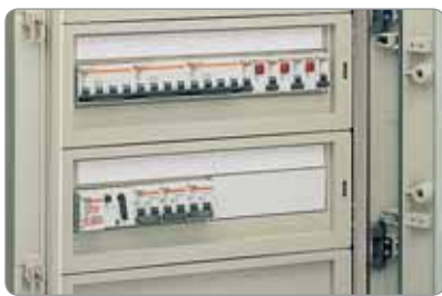
Detail from the circuit-marking system.
