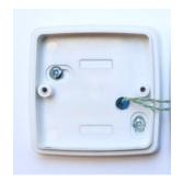
Now fix the face plate to the back plate using the screws provided.
