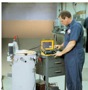
Measurement on a transformer in the workshop
