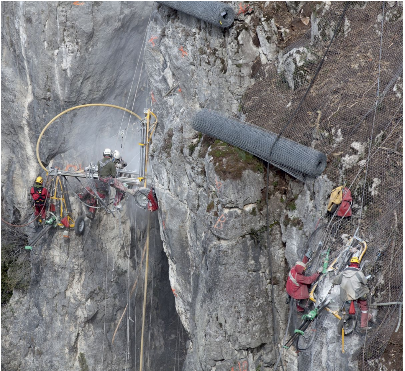
Hydrokarst, Voreppe, Isère France © Lafouche
