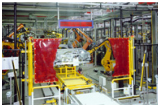
Classical muting solutions for body shell manufacture: Multiple light beam safety device with muting function, muting sensors, muting lamp and hinged flaps.
