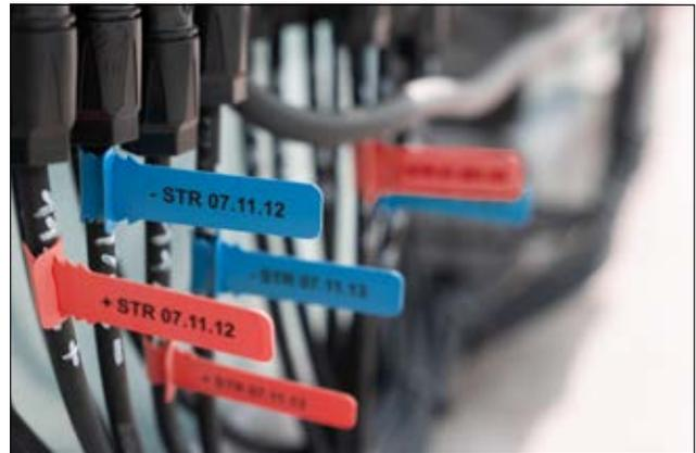
TAGPU LOOP - Cable marking solutions for labelling on the inverter.
