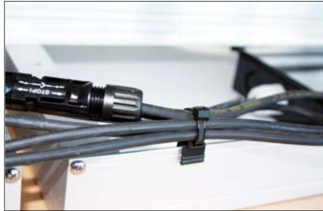
Easy module level cable management at the top of an edge.
