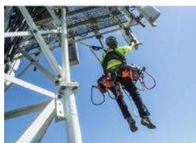
TETHER TOOLS AT HEIGHTS PREVENT DROPPED OBJECTS.
